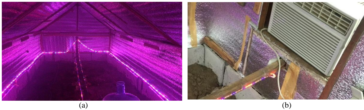
Fig. 7 (a) Lighting System and (b) Air-Conditioner Setup
