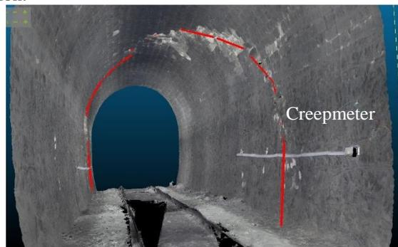
Figure 8 Fault zone in the Palu railway tunnel
