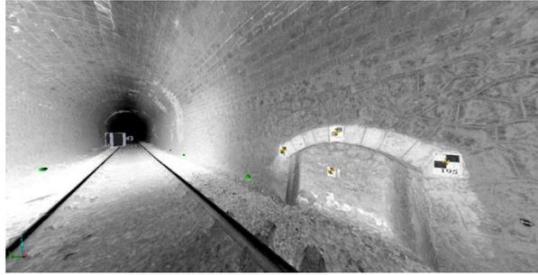
Figure 3 Control points in the tunnel
